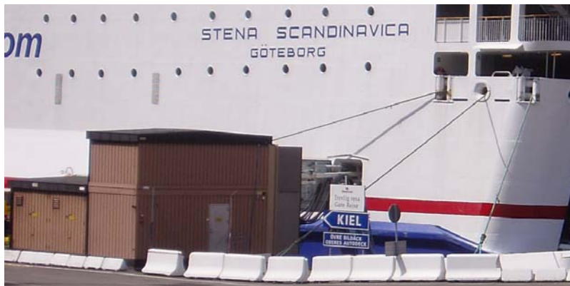
Figure 14 Shore to ship connections in the Gothenburg terminal
